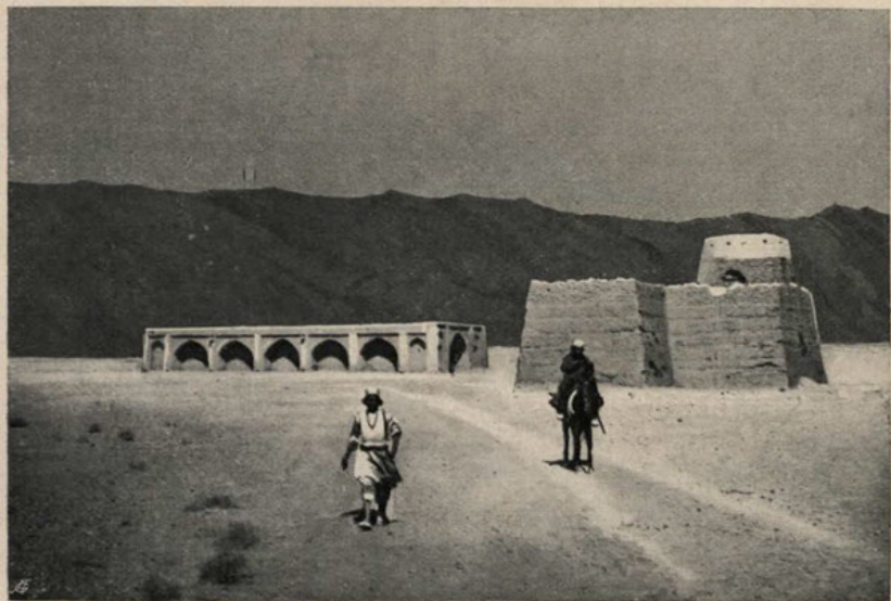
TYPICAL CARAVANSERAI AND MUD FORT IN THE DESERT BETWEEN YEZD AND KERMAN.
