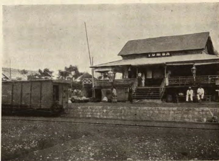
TUMBA STATION ON THE WEST COAST CONGO RAILWAY.
