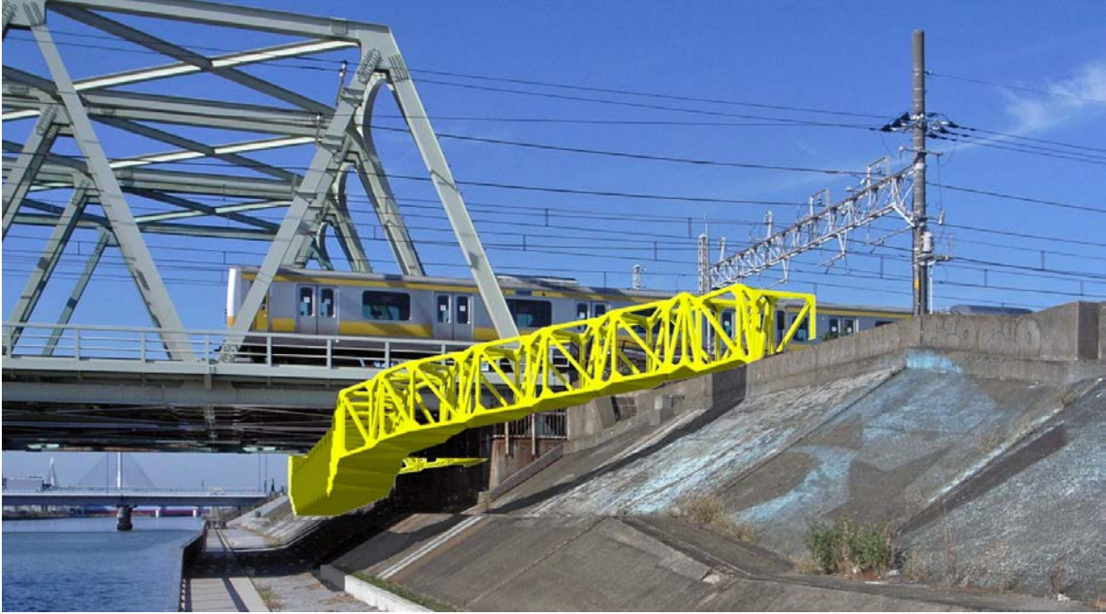
Figure 3: Visualization of retrofitting of a cycling/pedestrian path which continuity has been interrupted by a railway. The lightweight TZ could be partially suspended from the existing bridge. Without the necessity of heavy equipment, TZ is a feasible solution for countless situations.
