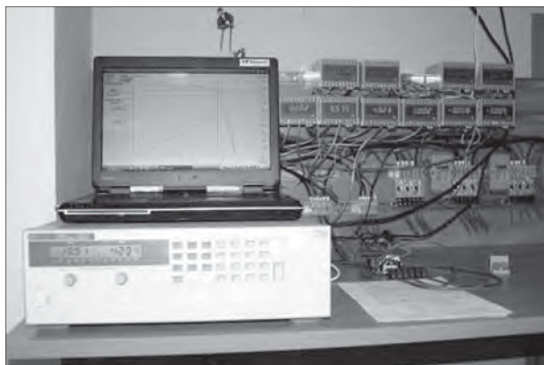
Fig. 1. The view of the E4350A simulator with the cooperating computer and roof modules' control desk.
