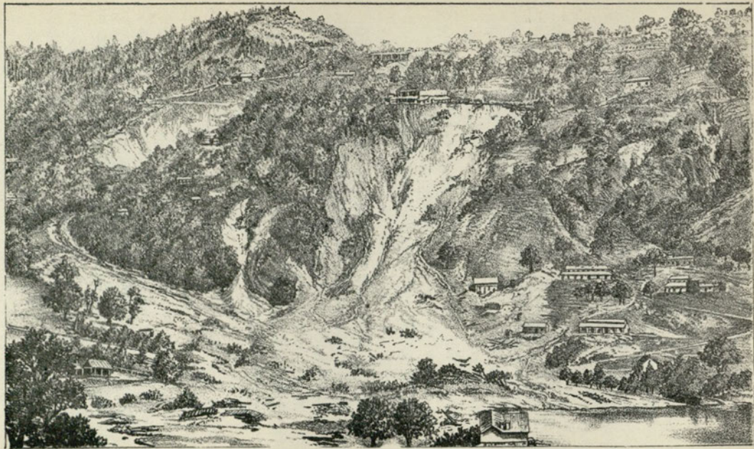
LANDSLIP AT NYNEE TAL.
