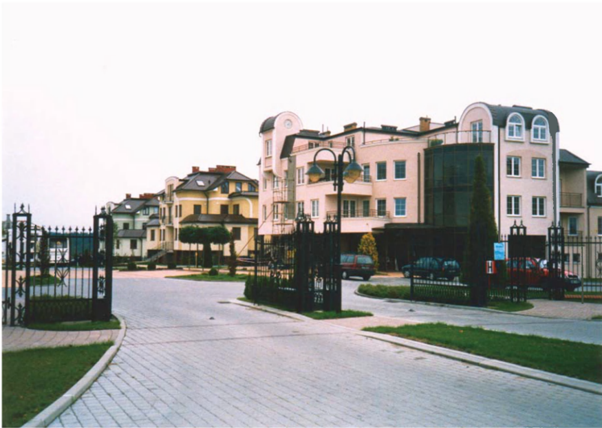
Photo 1. Gated community 'Osiedle Modre' in Straszyn near Gdansk, Poland, described in promotional literature as follows: 'Comfortable and stylish houses set in spacious building plots, flats with both garage and garden, fully landscaped grounds, modern technology, security and monitoring, perfectly planned communication system, separate access to each building plot, full telecommunications infrastructure, a sports and recreational complex with a horseriding club.'
