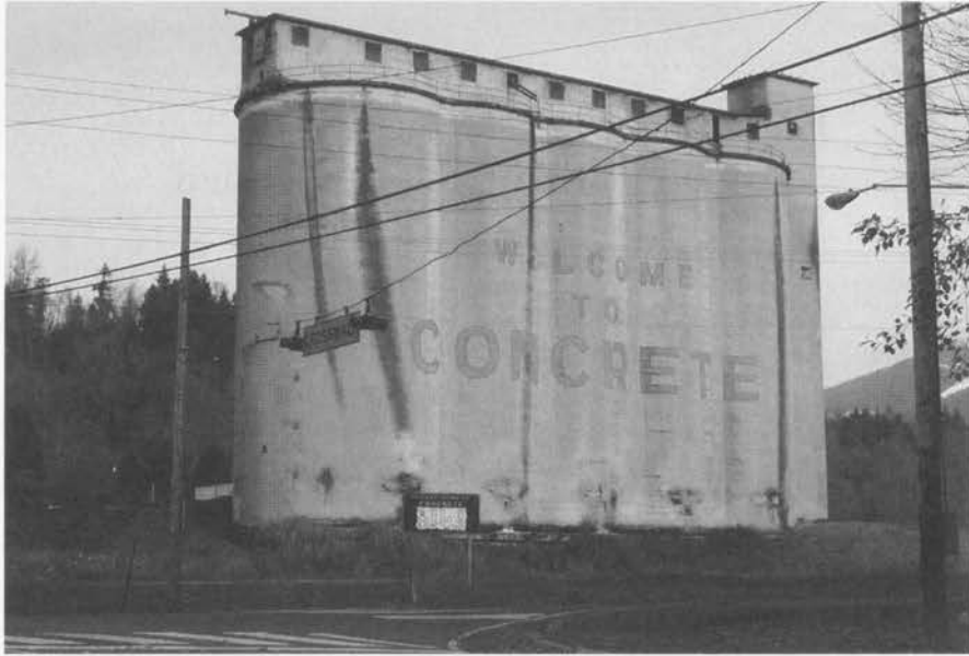
FIGURE 1. Abandoned cement silo in the town of Concrete, Washington, U.S.A.
