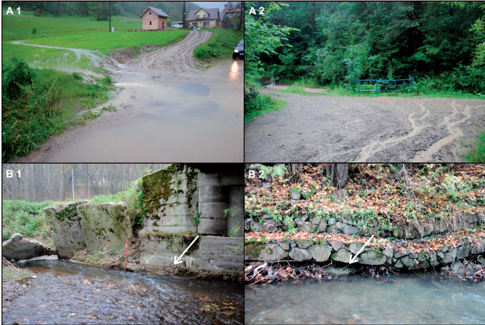
Figure 9. (A) Suspended sediment on the roads during heavy rainfalls: A1 – unused unpaved road, used unpaved road, paved road in the Jaszczce-Jamne catchment during continuous rainfall of 82 \text{ mm } 24 \text{ h}^{-1} in 15.05.2014, A2 – unpaved used road in the Homerka catchment during local downpour of 30 \text{ mm } 2 \text{ h}^{-1} in 28.07.2016, (B) River beds' position in relation to suspended bridgeheads and concrete structures: B1 – suspended bridgehead in the Uszwicka stream, B2 – suspended gabion in the Homerka stream
