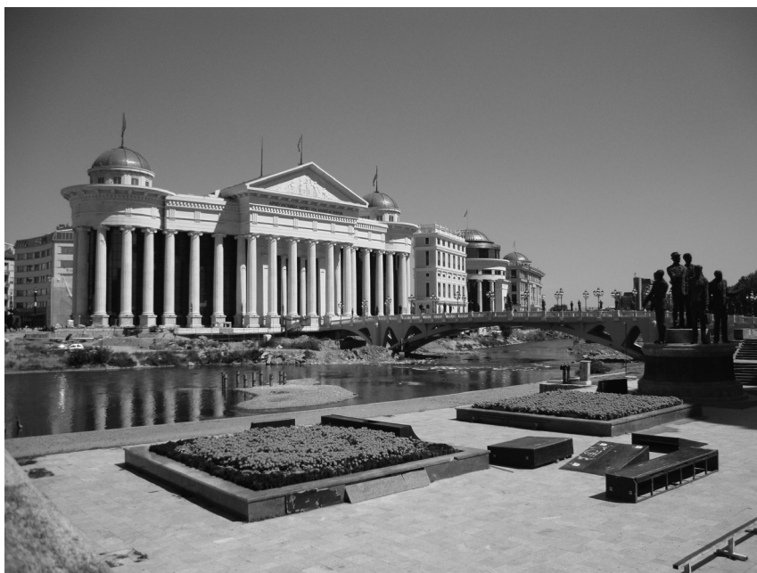
3. The building of the Court of Justice, state's archive and archeological museum (photo made by author on September 2013)
