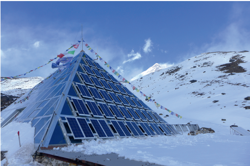
Figure 2. The almost 120 solar panels covering the pyramid form the most visible part of the complex system assuring the self-sufficiency of the station (by K. Janecka)
