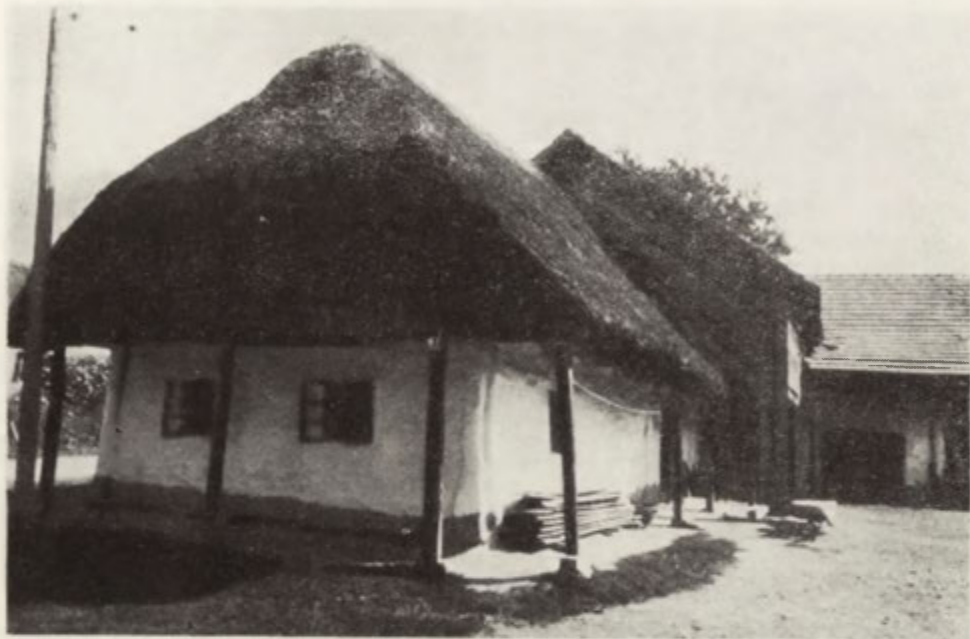
Fig. 3. An old type of farmstead with houses built „in a key”, first being a dwelling house, than the stable and the barn in the background
