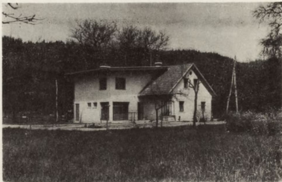
Fig. 8. A new modern urban house built in 1960. As the family do not pursue any farming, no farm buildings are attached to the house
