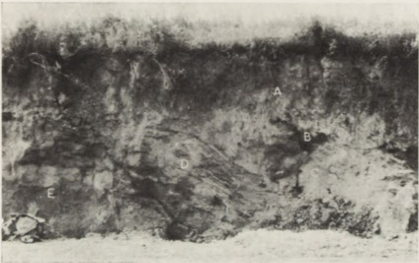
Fig. 7. Road tunnel south of the Gorzyczanka valley
