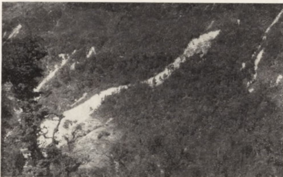
Plate 9. Great landslide on the forested slope near Poobong (photo taken 24 Dec. 1968)
