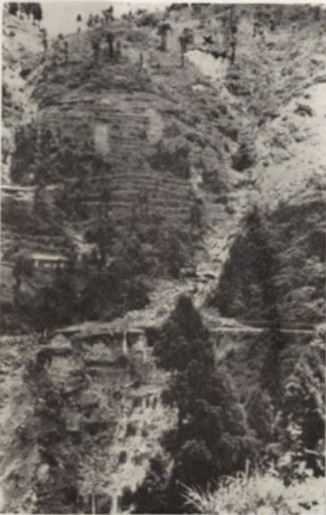
Plate 21. Complex debris flow crossing the road Ghoom - Darjeeling. Result of heavy rain in June 1950 (photo Das Studio, Darjeeling)
