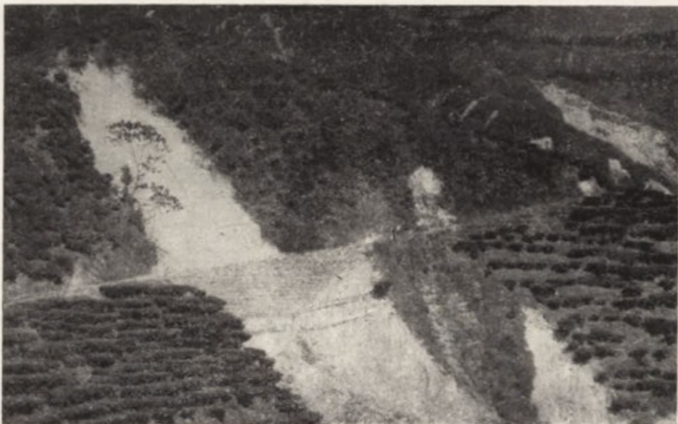
Plate 7. Mudflow created on artificial undercutting near garden road at Poobong T.E. (photo taken 24 Dec. 1968)
