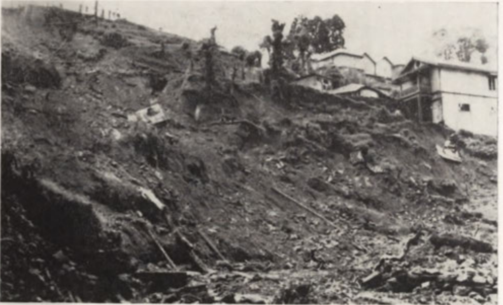
Plate 20. Big landslides in the the centre of Darjeeling after heavy rain in June 1950 (photo Das Studio, Darjeeling)
