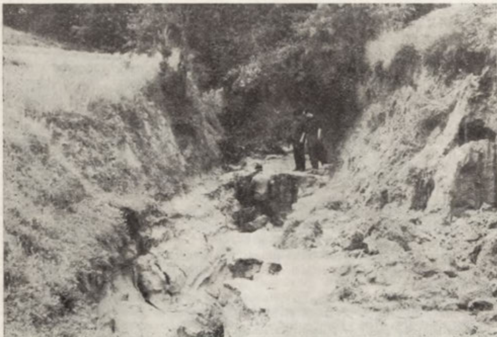
Fig. 8. Dirt road gap, eroded during heavy rainfall; situated in the loess area of the Lublin Plateau. Photo by S. Ziemnicki
