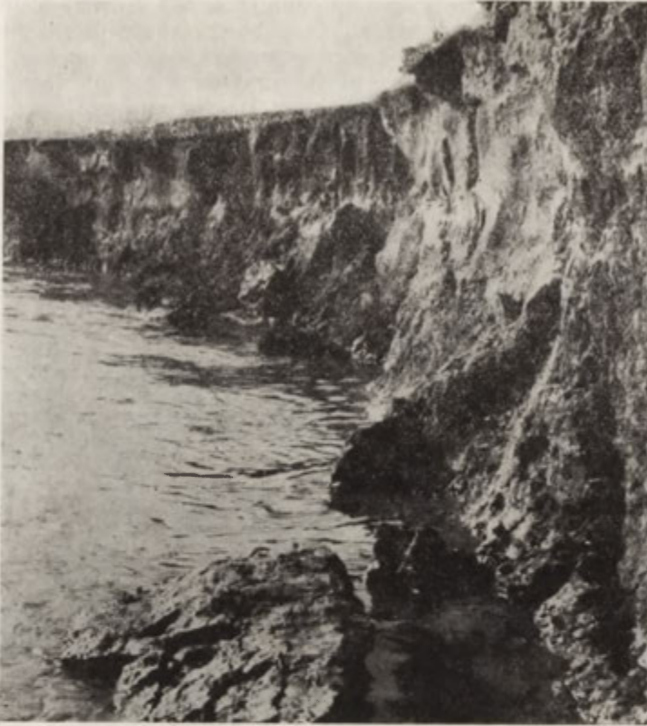
Fig. 8. Krajowice. At the raised water-stage there is intense bank slumping. Mada blocks falling to the bed are gradually washed away by the water (Photo K. Klimek, Febr. 1972)
