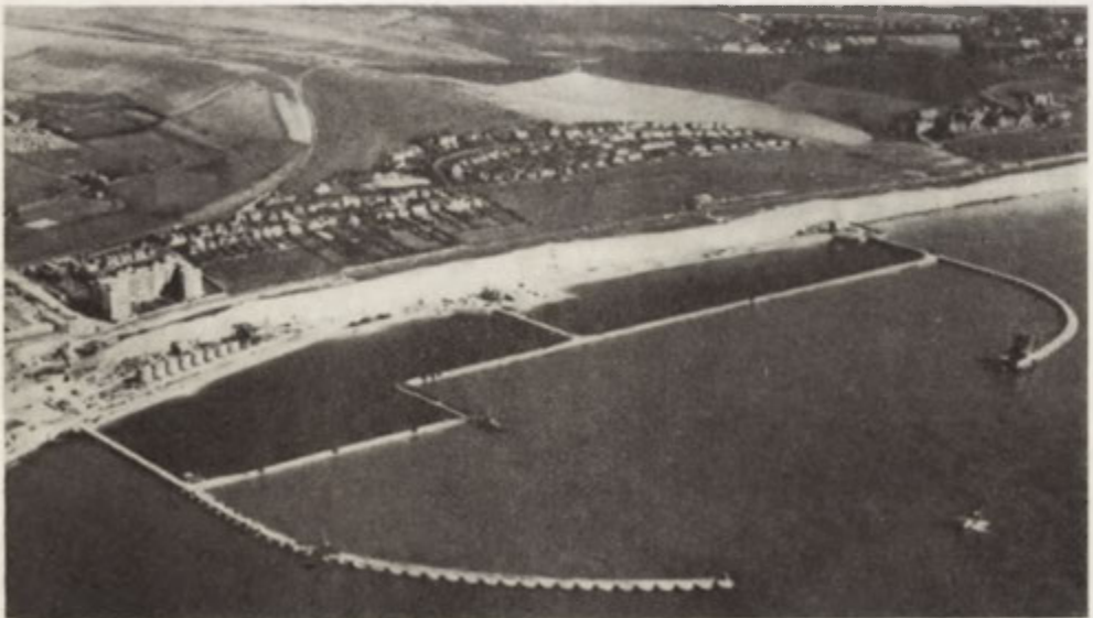
Fig. 3. Brighton Marina, southern England: a stage in coastal reclamation and the construction of breakwaters
