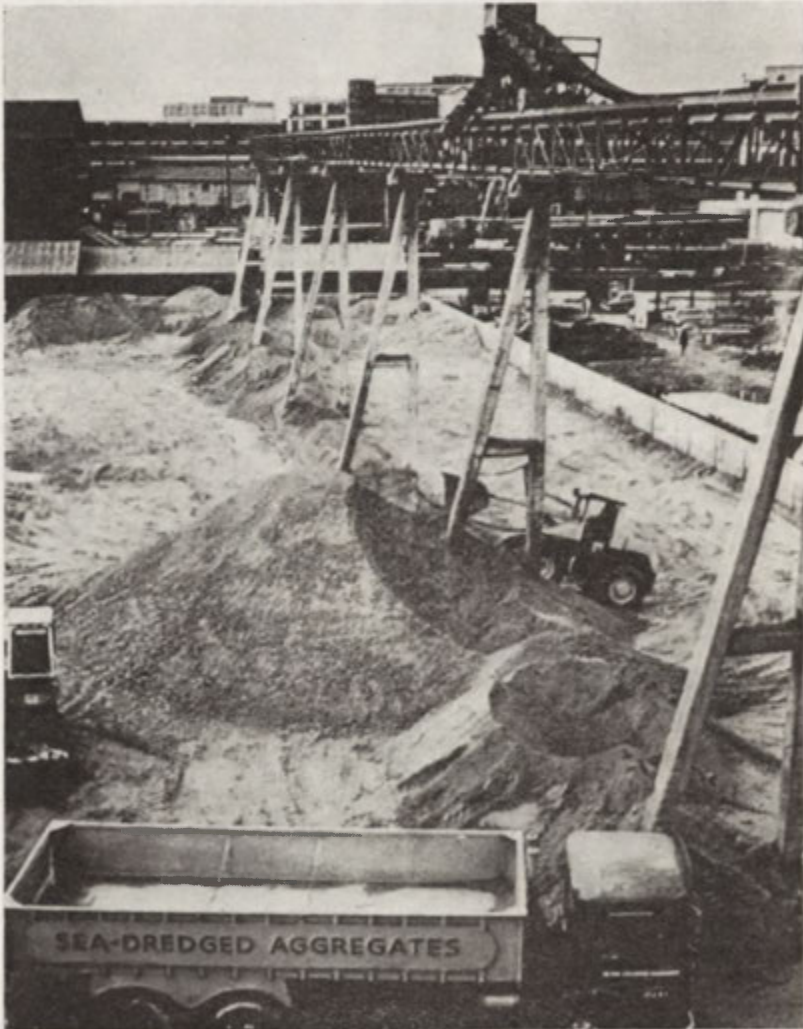
Fig. 9. Marine aggregate plant, Port of London, England: one of many such plants handling offshore dredgings
