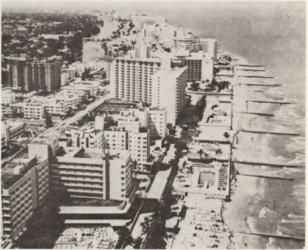
Fig. 4. Miami Beach, Florida: an amenity-recreational complex requiring defences against coast erosion and flooding
