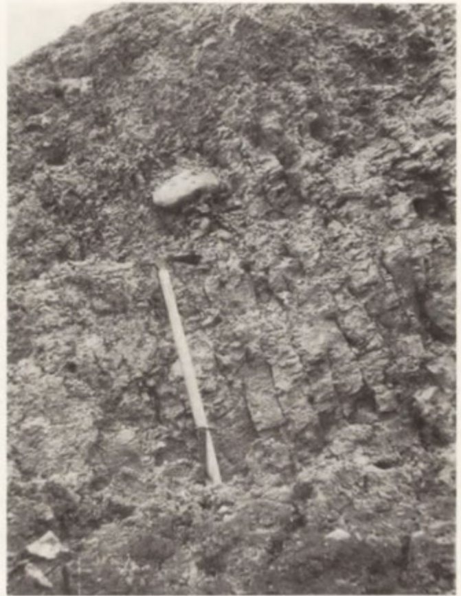
Fig. 7. Fragment of interior structure of clay wall (Photo by J. Szupryczyński, July 1963)
