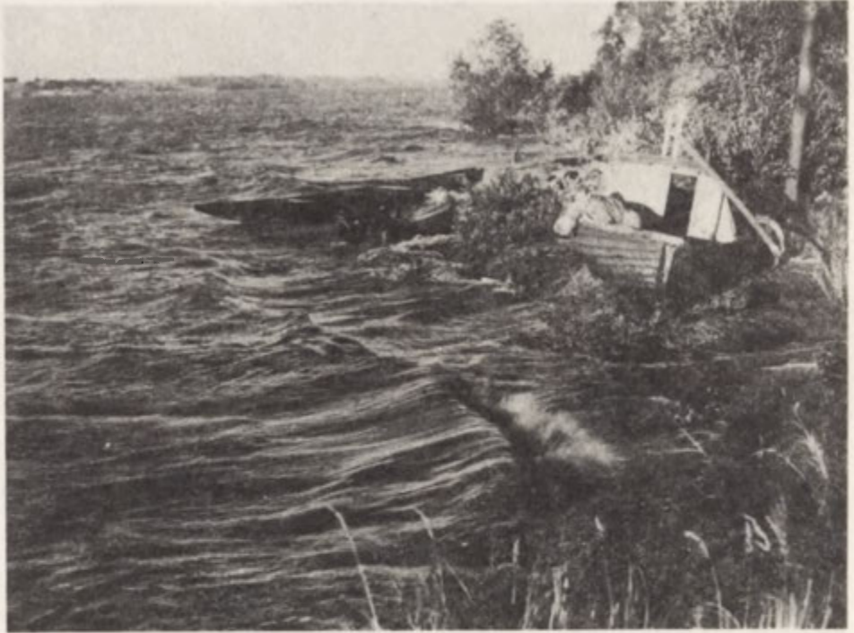
Photo 1. Dobięgniewo. Low bank destruction by waves at high water stage in the reservoir. Wave height up to 50 cm, 21st August 1980
