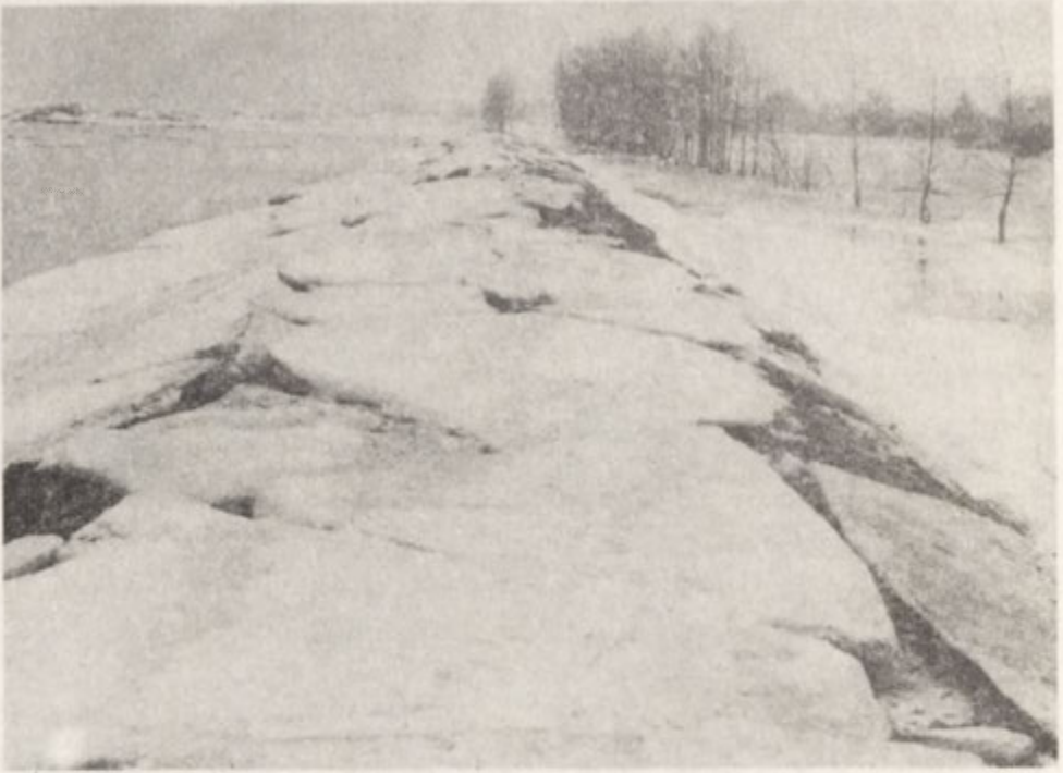
Photo 7. Ice floe on the embankment, three weeks after the maximum water level during the catastrophic flood in Jan. 1982
