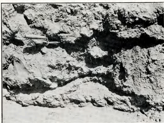
C. Cross section showing floor level. Photographs by Wesley Bradfield.
