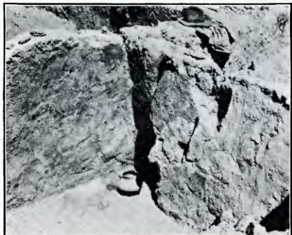
A. Adobe brace for weak wall.
