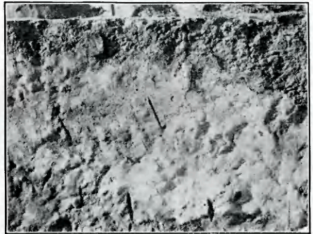
D. Plaster on wall.
