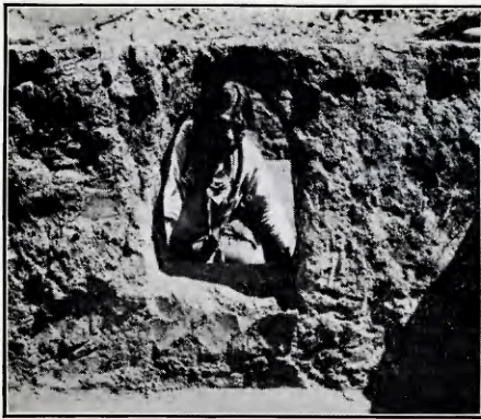
C. Oval-topped doorway.
