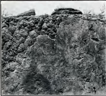
A. Wall construction, showing nodules.
