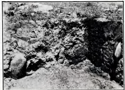
F. Cobblestone foundations.
