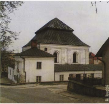
Photo 3. Old synagogue in Szczepieszyn (Eastern Poland)
