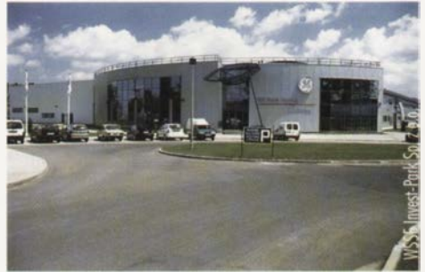
Photo 3. General Electric Power Controls in Kłodzko (Lower Silesia)
