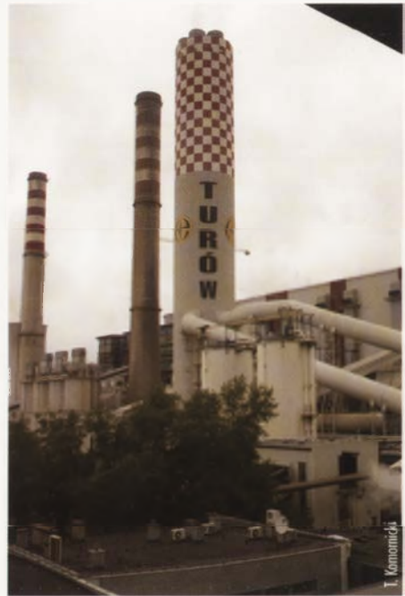
Photo 1. Turoszów power plant (based on lignite) with new sulphur scrubbers
