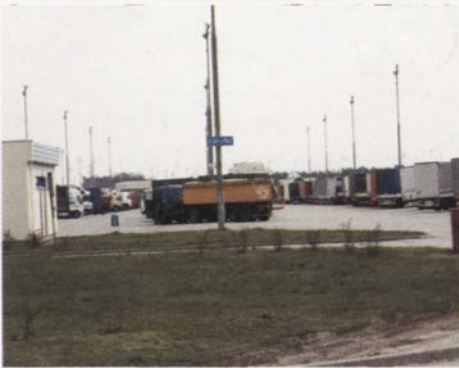
Phot. 5. Customs terminal in Świecko, through which hundreds of trucks pass every day, entering Polish road network
