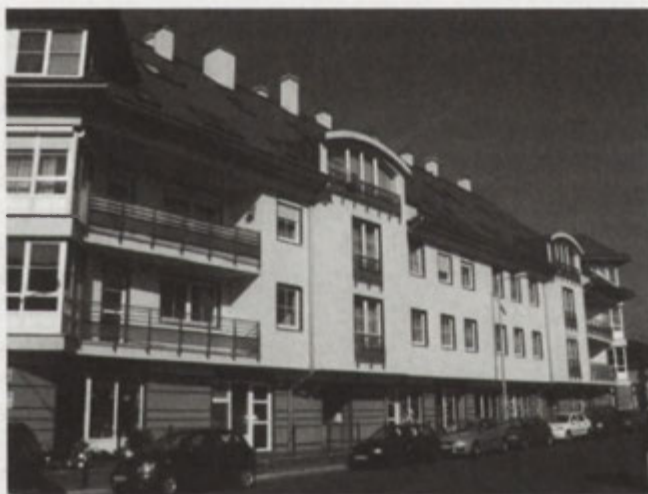
Photo 4. Brand new residential building in Újpest-Centre
