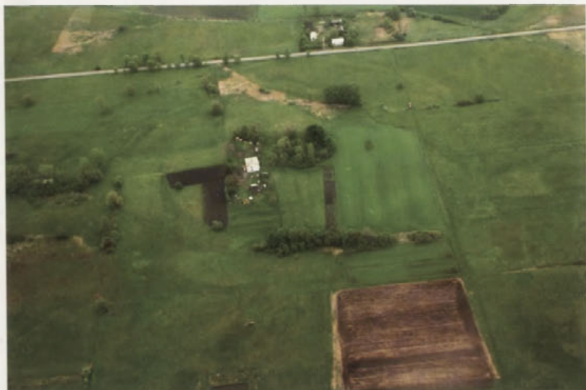
Fig. 2. Busówno, Wierzbica commune, Chełm district, site 1. Aerial view of the stronghold from the western side (photo by K. Trela)
