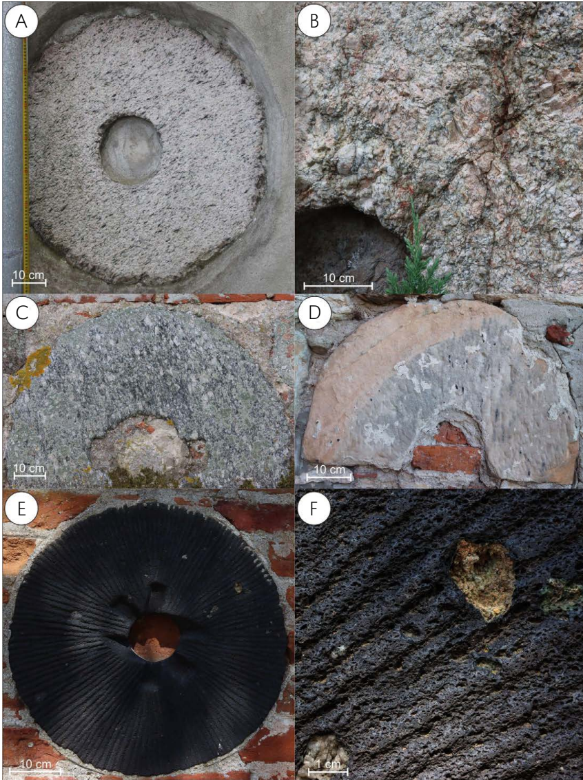
Figure 4. Millstones in church walls; A - millstone or semi-finished product in Bodzanów in Mazovia, leucocratic gneiss (erratic), B - semi-finished product at the entrance to the church in Kraskowo (Masuria), coarse crystalline pegmatite (erratic), C - worn millstone or semi-finished product in Rogiedle (Warmia), gneiss with small crystals (erratic), D - semi-finished product used as building material in the monastery church in Sulejów, sandstone from the vicinity of Wąchock (northern Mesozoic margin of the Holy Cross Mountains), E, F - worn millstone in the ruins of the church in Wocławy in Żuławy, porous volcanic rock, most likely imported from the Eifel massif (?). (Photos by P. Czubla)
