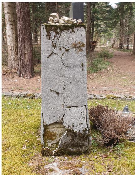
Fig. 2. Monument in Tylawa, side view with visible cracks, April 2022, M. Saryusz-Wolska.
