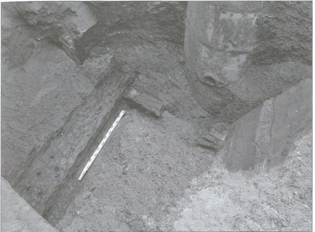
Fig. 13. Kołobrzeg, Armii Krajowej street. Water circuit connection and the sewage canal. Photo by B. Wywrot-Wyszkowska.
