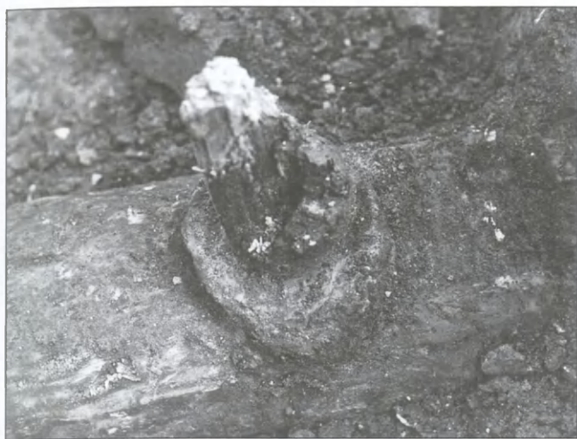
Fig. 9. Kołobrzeg, Plot 29 Narutowicza street. Fragment of the water conduit with remains of the vertically installed pump. Photo Z. Polak.
