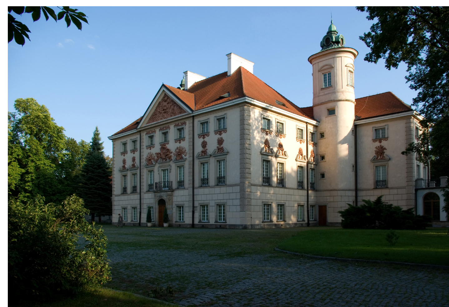
Fig.1. The Bieleński Palace in Otwock Wielki, near Warsaw.
