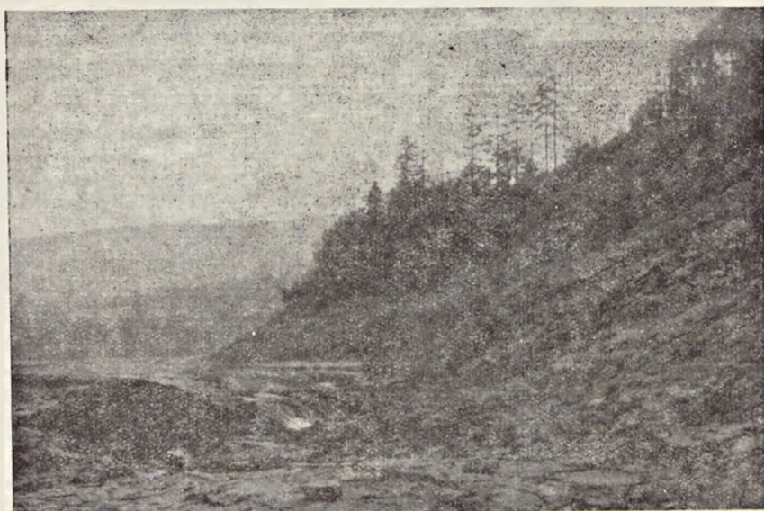
Fig. 1. Steep western bank of the reservoir at Porąbka
