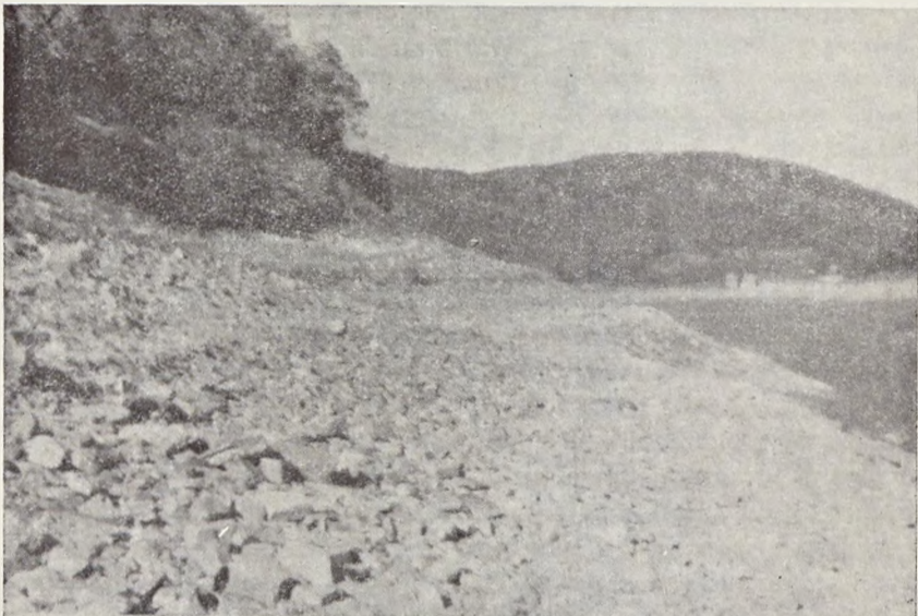
Fig. 3. Configuration of the bank of the middle part of the reservoir at Porąbka
