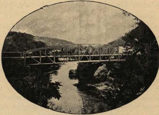
Vrbasbrücke in Banjaluka.
