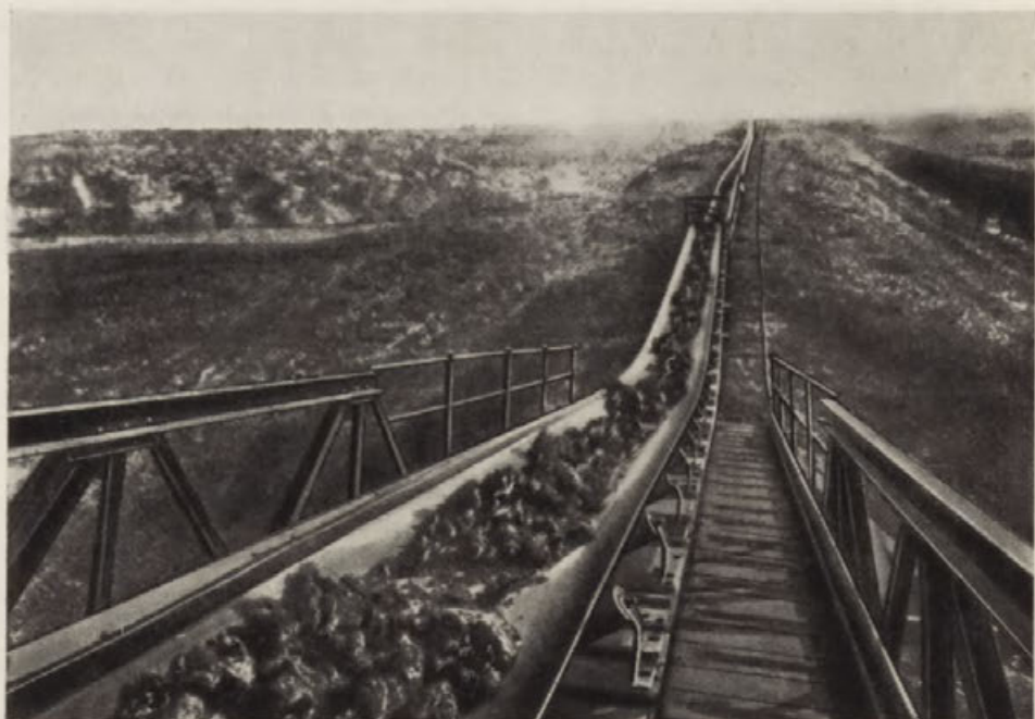
Fot. 2. Transport surowca z kopalni do zakładu w cegielni Stewartby The transport of raw material from the clay pit to the brick works in Stewartby
