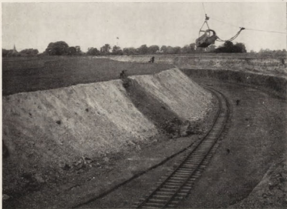
Fig. 4. Opencast ironstone quarry ("Type 2") in Rutland "Walking dragline" removing overburden of about 12 m. creating level surface behind quarry, instead of "hill-and-dale", with speedy agricultural restoration
