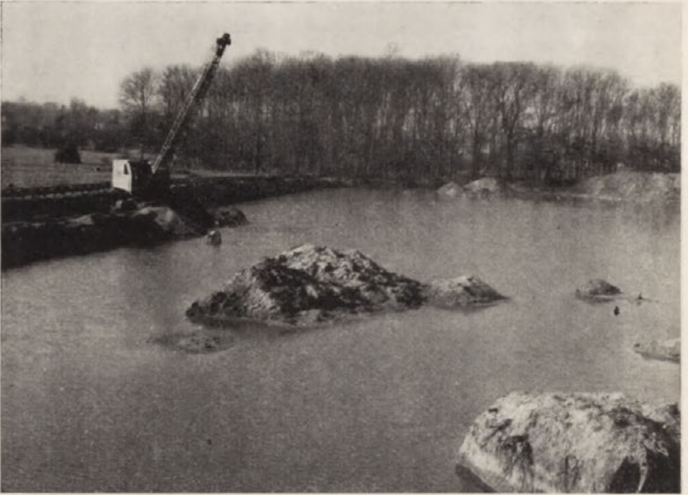
Fig. 6. A "wet" gravel pit in Leicestershire ("Type 4") Dragline excavator digs gravel from beneath water
