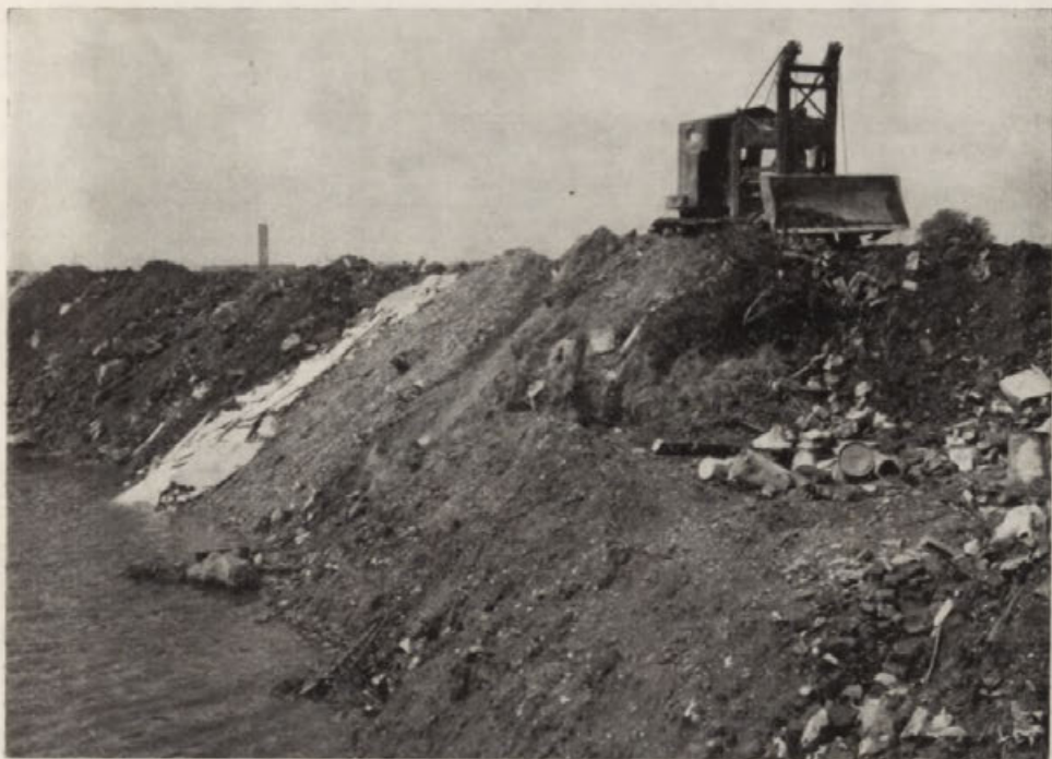
Fig. 7. Filling a disused "wet" gravel pit, ("Type 4") in Hertfordshire The debris is dumped by lorries and bulldozed into the water
