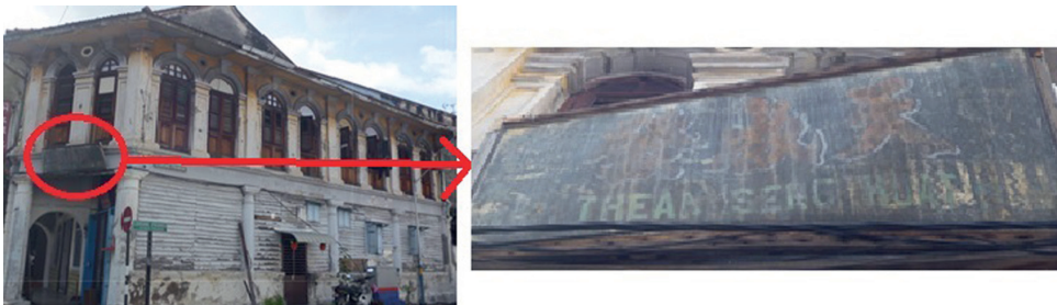
Figure 6: Thean Seng Huat — the building housing the shop and the first shop sign (circled)
