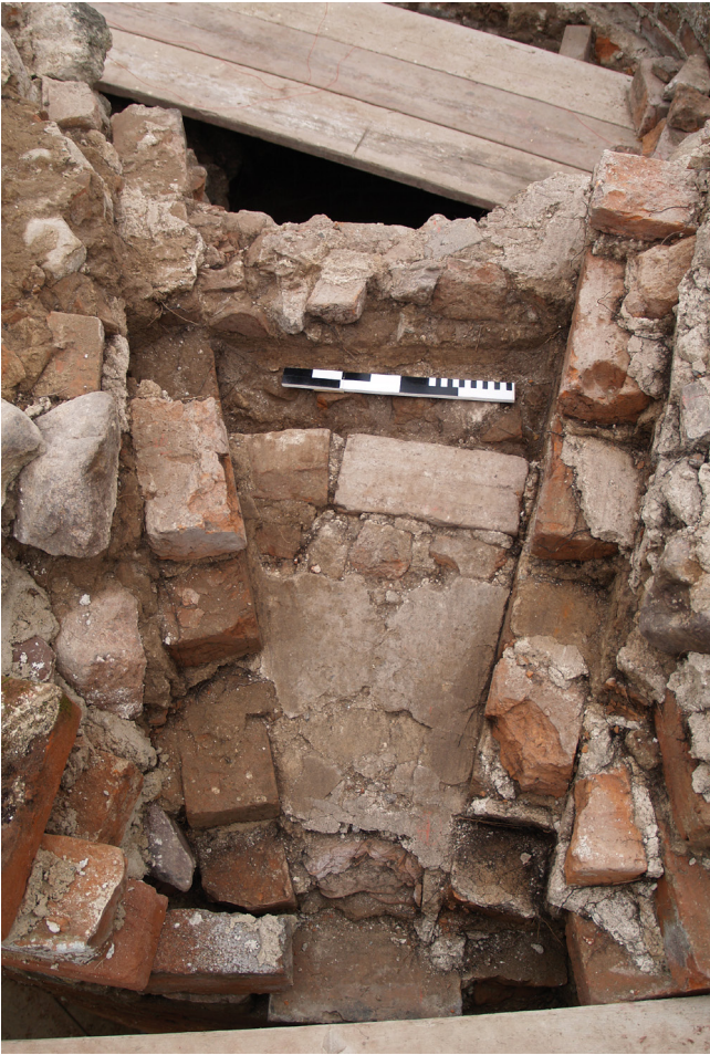
Fig. 7. Greiffenberg (Brandenburg), gun loop on the corner tower. Photo C. Krauskopf, BLDAM.
