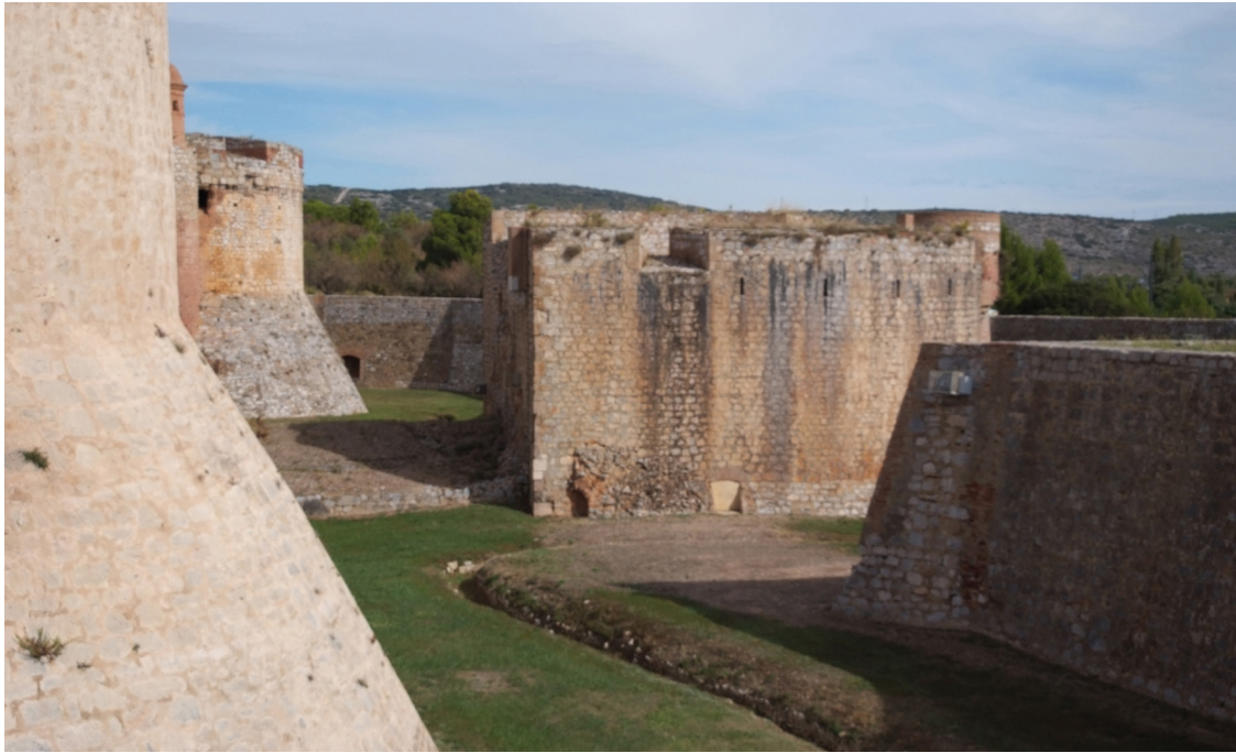
Fig. 18. Salses (Pyrénées orientales), 1497: ditch, caponier and corner towers with talus added after failed French siege 1503. Photo P. Purton.
