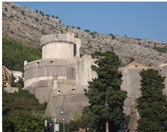
Fig. 17. Dubrovnik (Croatia). Minčeta tower and surrounding outer wall and curtain rebuilt by Michelozzo from 1461. Photo P. Purton.
