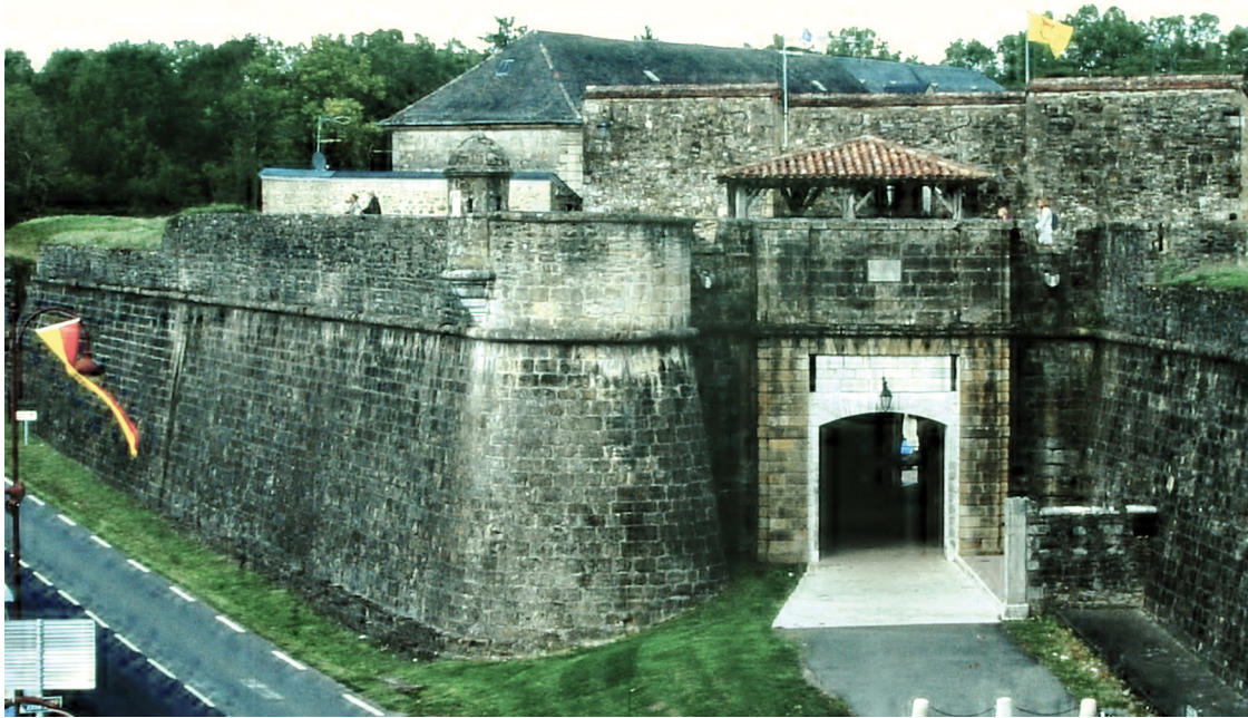
Fig. 20. Navarrenx (Pyrénées Atlantiques), bastion fortress built by Italian engineer 1530s. Photo P. Purton.
