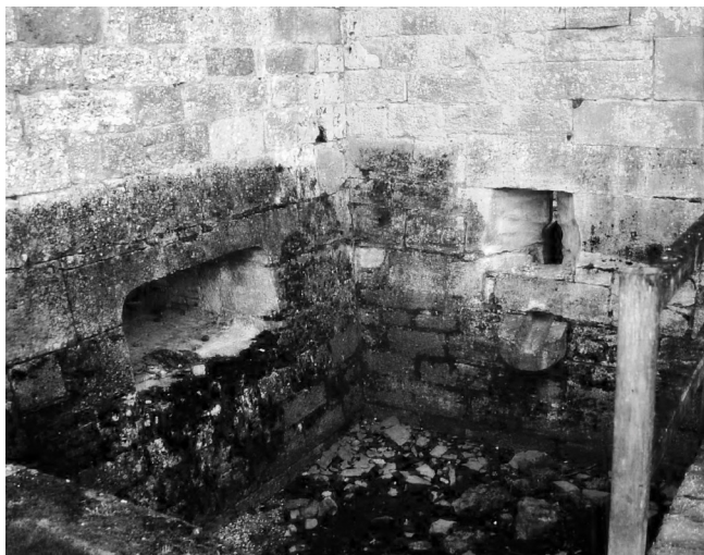
Fig. 15. Auxonne (Côte d'Or). Embrasure in the foot of the gun tower, covering ditch and entrance. Photo P. Purton.
