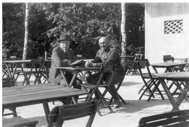
Fig. 4. Albin Jura and Captain Stanisław Koźmiński during the construction of the Piłsudski Mound in Sowiniec (Cracow). Information overleaf: 'Capt. Koźmiński and A. Jura, spring 1936'. Photo from the Archive of the Department of the Palaeolithic and the Mesolithic, the Archaeological Museum of Cracow.
