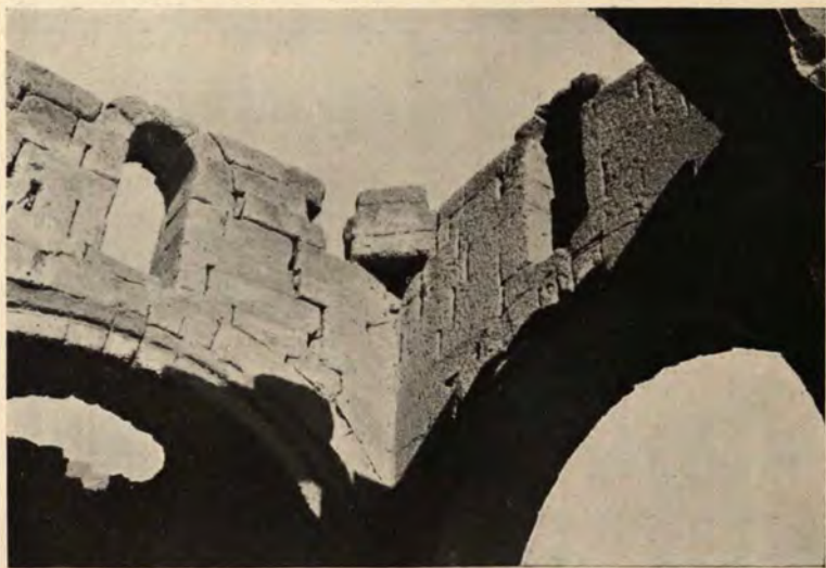
FIG. 221.—TOMARZA, CHURCH OF THE PANAGIA, SETTING OF DOME.
