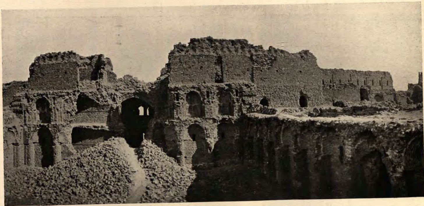
FIG. 91.—UKHEIDIR, COURT D AND NICHED FAÇADE OF THREE-STOREYED BLOCK.
