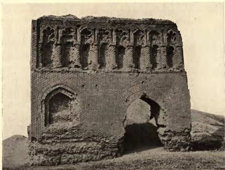
FIG. 43.—RAQQAH, BAGHDÂD GATE FROM EAST.
