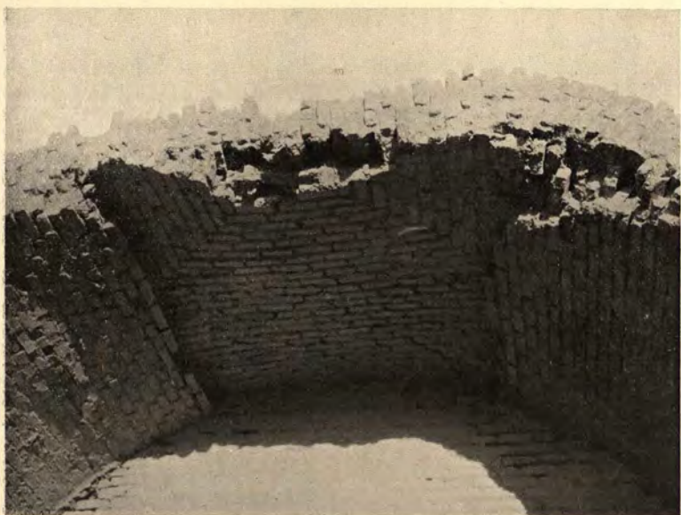
FIG. 132.—KHÂN KHERNÎNA, DETAIL OF FLAT VAULT.
