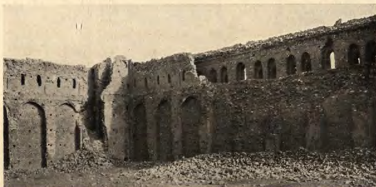
FIG. 84.—UKHEIDIR, STAIR AT SOUTH-EAST ANGLE.
