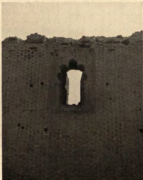
FIG. 142.—SÂMARRÂ, RUINED MOSQUE, WINDOW IN SOUTH WALL.
