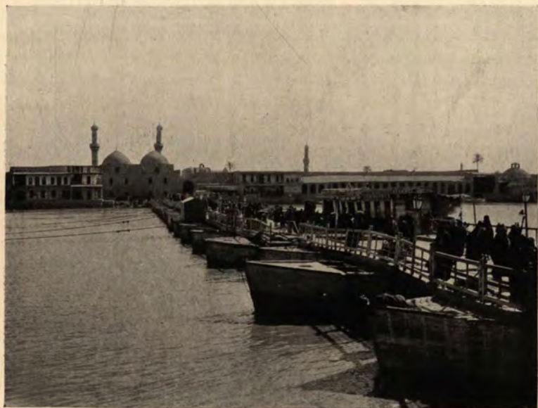
FIG. 111.—BAGHDÂD, THE LOWER BRIDGE.
