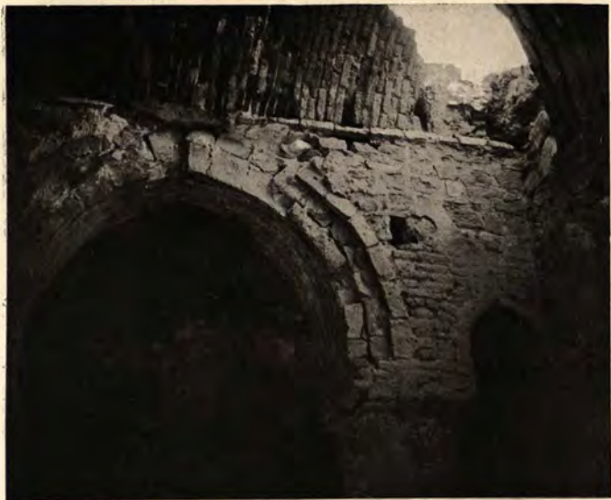
FIG. 92.—UKHEIDIR, VAULT OF ROOM I.
