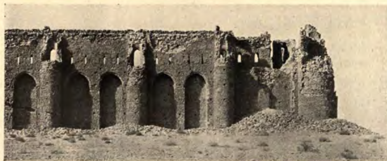
FIG. 83.—UKHEIDIR, NORTH-EAST ANGLE TOWER.
