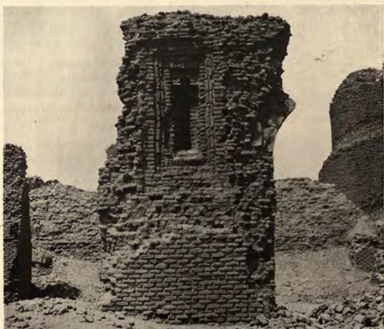
FIG. 166.—ABU DULÂF, NICHED PIER OF NORTHERN ARCADE.
