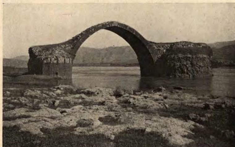
FIG. 186.—JEZÎRET IBN 'UMAR, BRIDGE.
