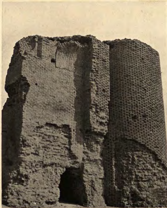
FIG. 141.—SÂMARRÂ, RUINED MOSQUE, SOUTH-WEST ANGLE TOWER.
