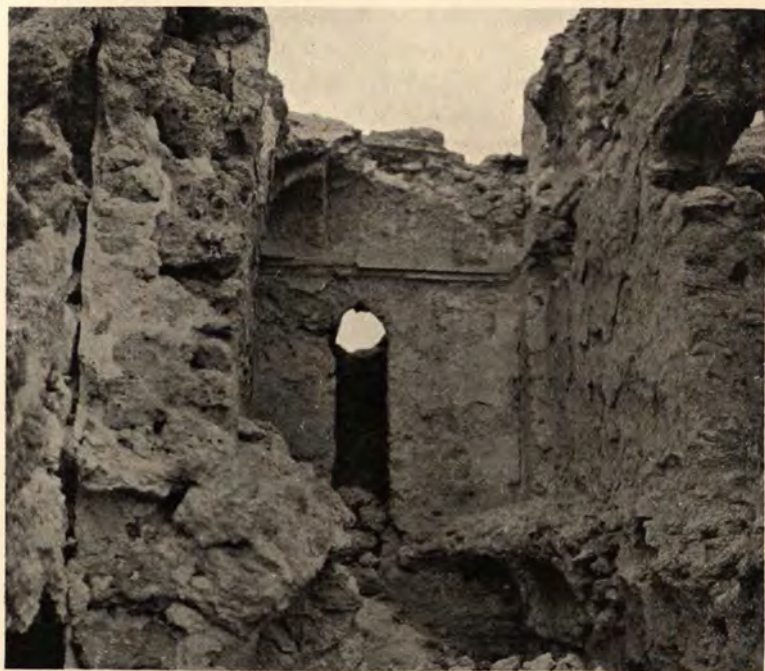
FIG. 74.—BARDAWÎ, EAST END OF VAULTED HALL.
