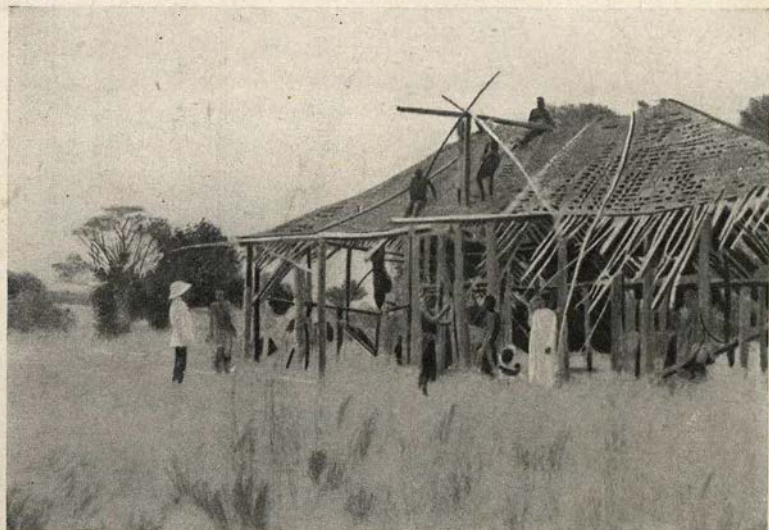
HOUSE CONSTRUCTION IN UGANDA
