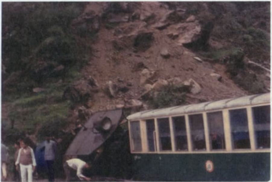
Subsiding Hill-Cart Road at lower Pagla jhora and damage to a railway engine at upper Pagla jhora by large rolled boulders.
